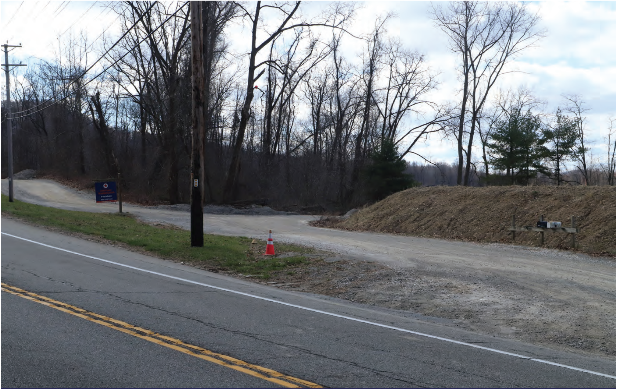
Photo 21 - NY Rte. 9 near Century Aggregates Quarry Entrance EXISTING CONDITION
