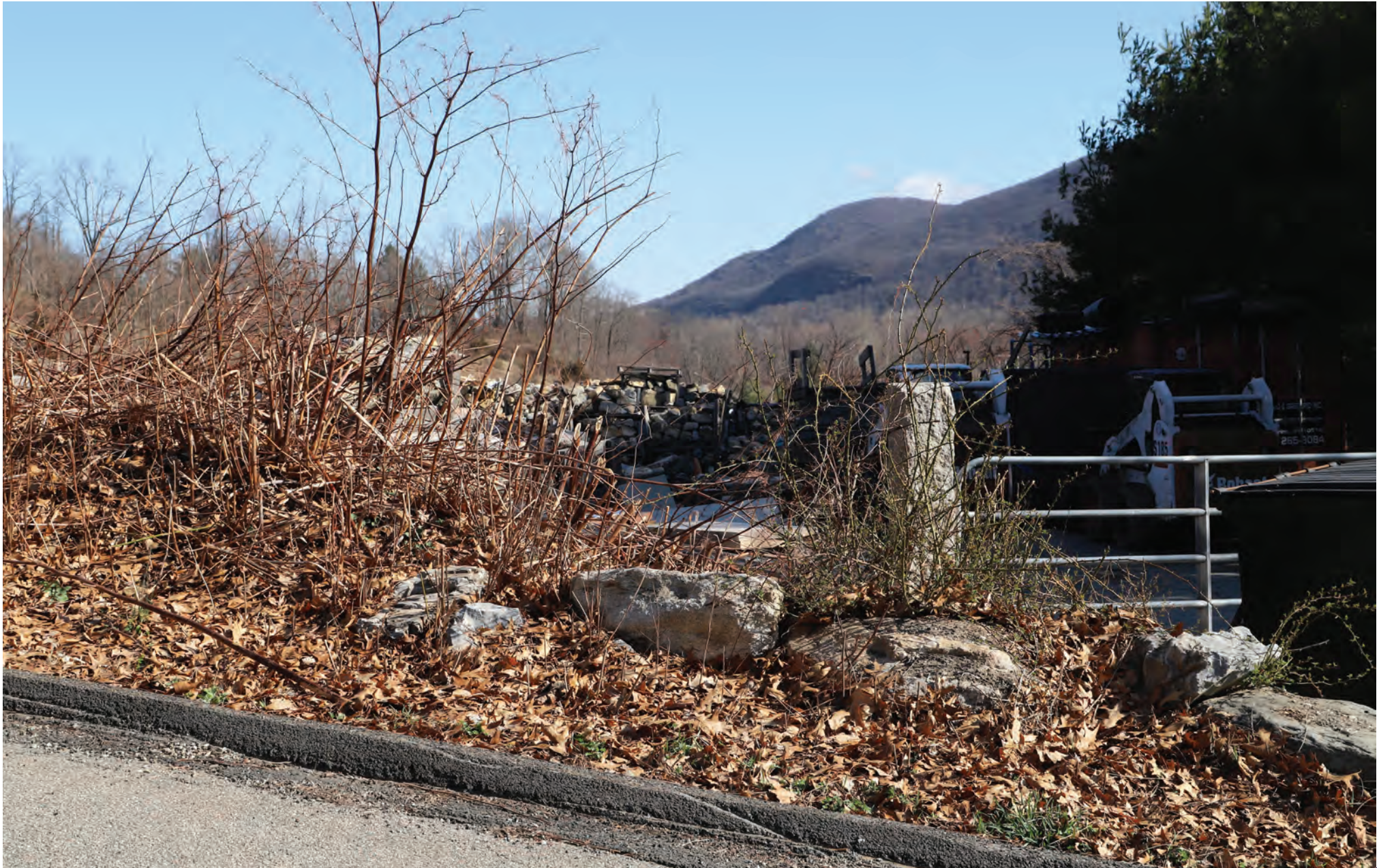
Photo 02 - Skyline Dr near NY Rte 9 EXISTING CONDITION
