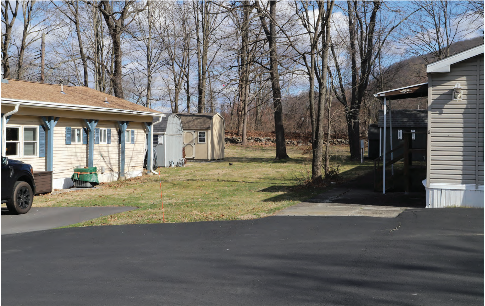
Photo 11 - Baseline Rd near #9 EXISTING CONDITION
