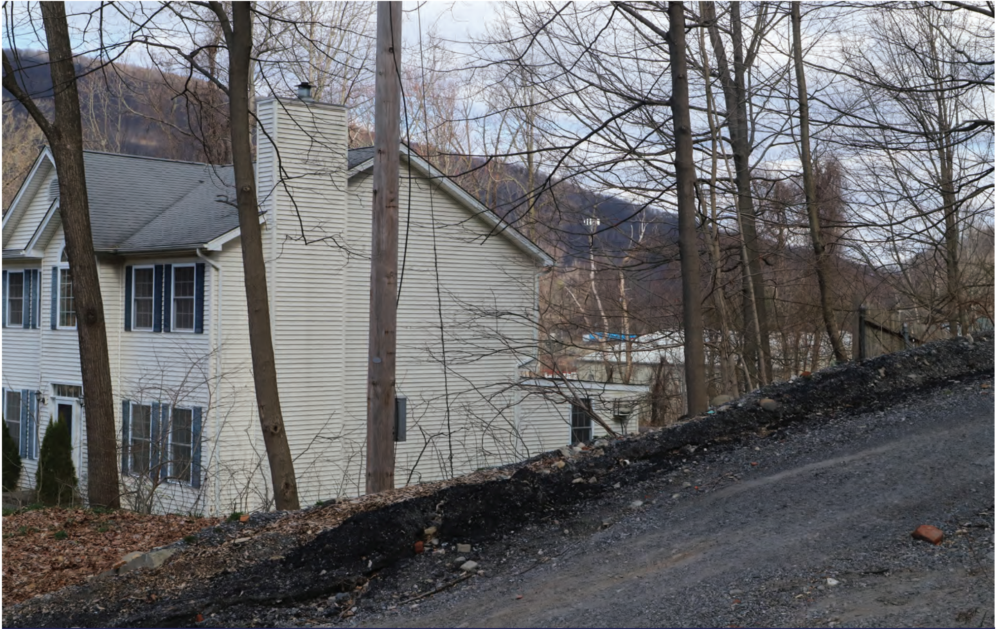
Photo 13 - Carol Ln near #252 SIMULATED CONDITION
